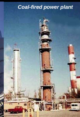
Coal-fired power plant
