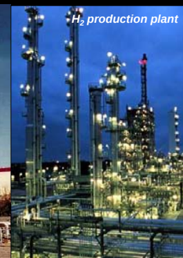
H 2 production plant
